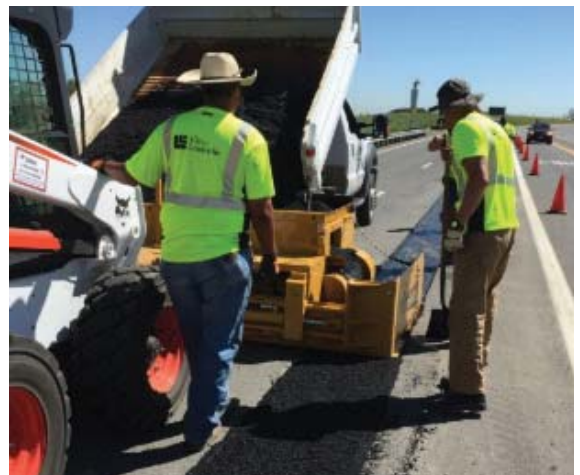
"Mill and fill" has never been easier.
